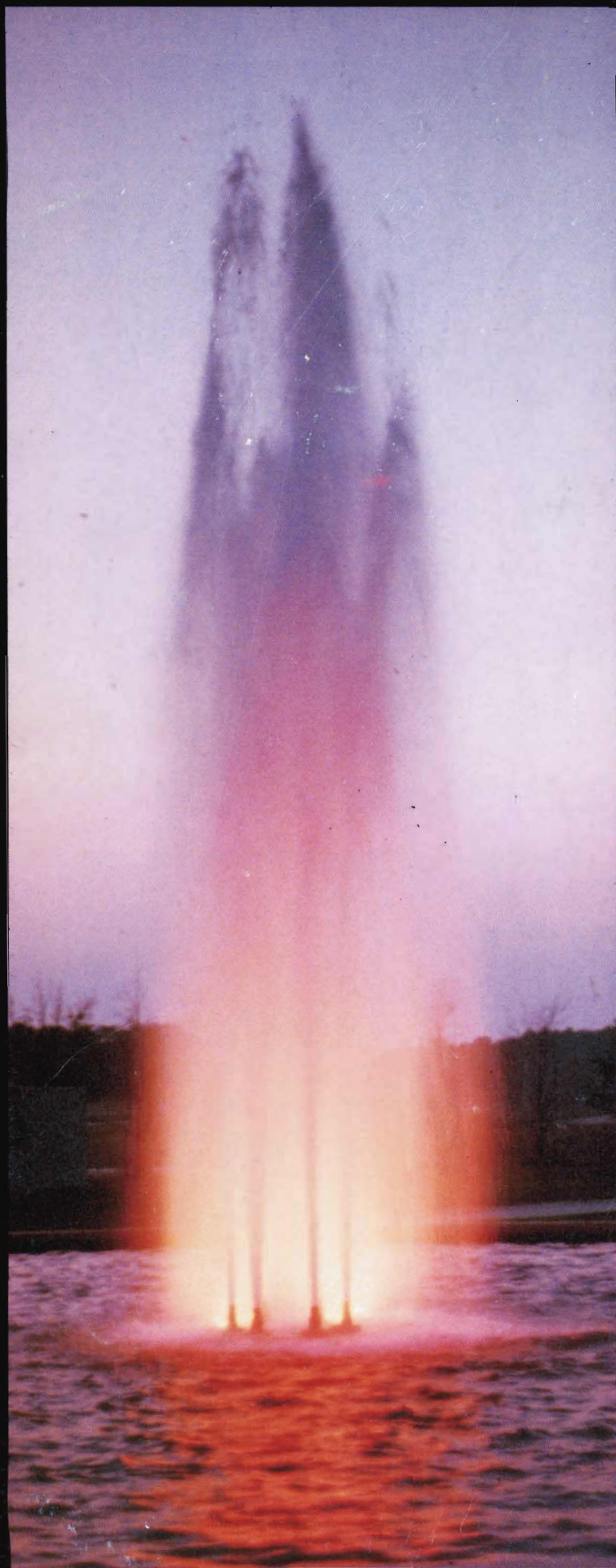
A typical installation where a cluster of aeration nozzles is used effectively as a heat-exchanger on air conditioning systems.
