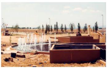
The entry fountain at the Sandia Casino is designed to appear much like a natural pond. The fountain incorporates three large Oase C-Line nozzles on flanged standpipes. The casino has a variety of nozzles such that the fountain effect can be varied over time. A wind control sensor is utilized to prevent the fountain spray from wetting the entry area.
